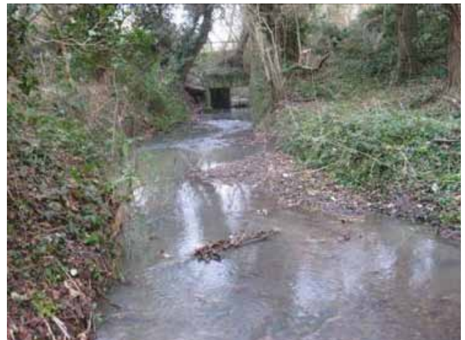
Improved channel conditions resulting from mitigation measures outlined above.
